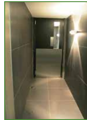
New walkway from the foyer to the kitchen.
